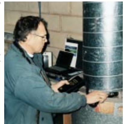
Spraybooth emissions monitoring
